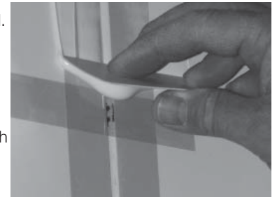
FIGURE 17: APPLYING THE PAINTER TAPE HORIZONTAL IN 3' SECTIONS
