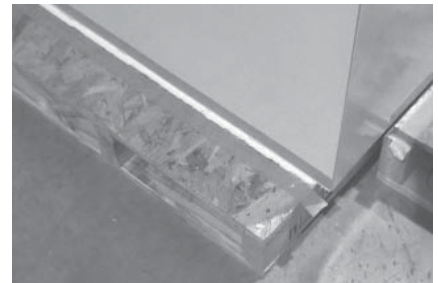
FIGURE 22: HORIZONTAL SEAM FILLED COMPLETELY WITH SEALANT
