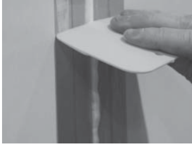
FIGURE 18: REMOVING EXCESS SEALANT
