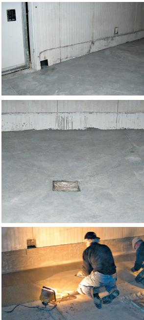
Flooring installed in a blast freezer of a food manufacturing plant quickly deteriorated and needed to be replaced one year after installation. The original protection system did not withstand sudden changes in temperature caused by hot water washings. Cracks appeared around the floor drains allowing water infiltration under the coating causing the surface to flake and breakdown.
