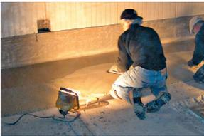
Flooring installed in a blast freezer of a food manufacturing plant quickly deteriorated and needed to be replaced one year after installation. The original protection system did not withstand sudden changes in temperature caused by hot water washings. Cracks appeared around the floor drains allowing water infiltration under the coating causing the surface to flake and breakdown.
